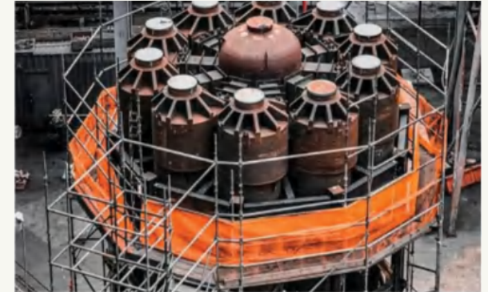
FCCU internals | Critical shutdown work
